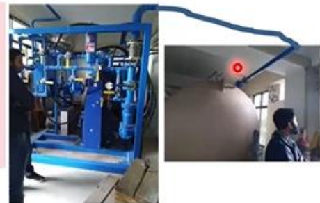
Highly insulated SF6 Gas: Transfer setup
